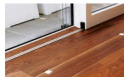
Sliding track, discretely installed into floor.
